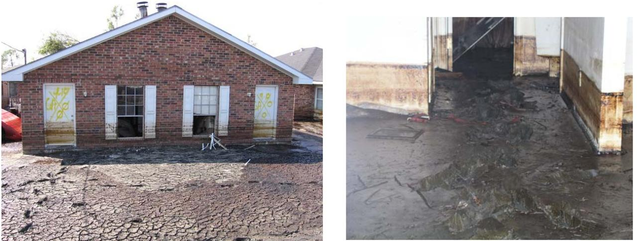
Figure 1: Photographs showing heavy oil deposits and staining on the exterior and interior of some homes.
