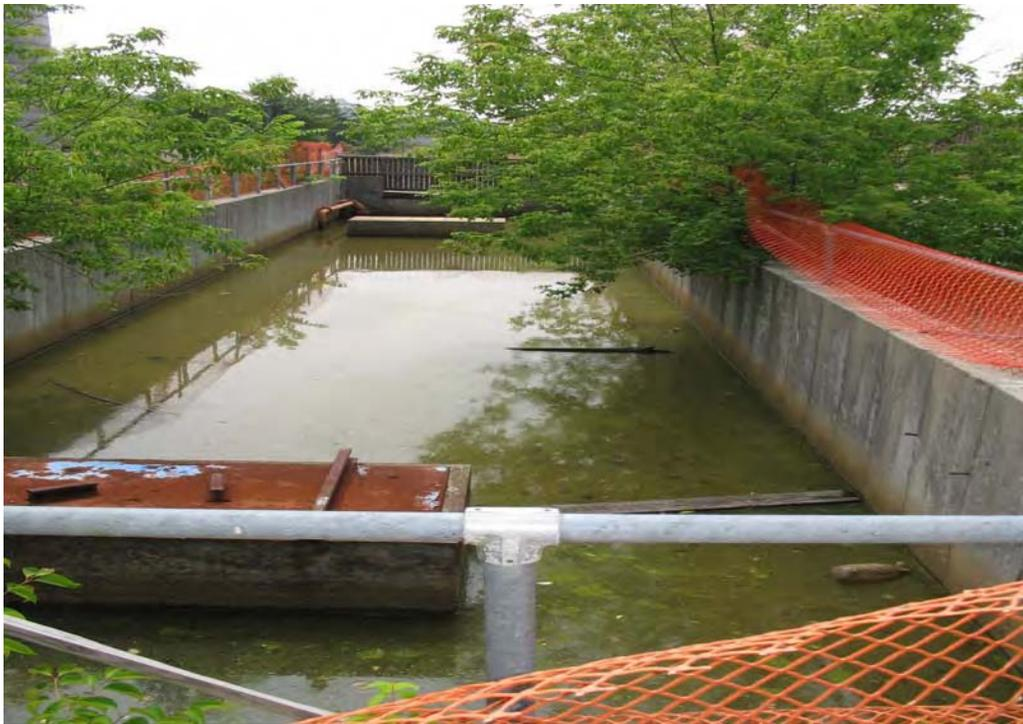
Picture 4: Lagoon in the Dricon process area
