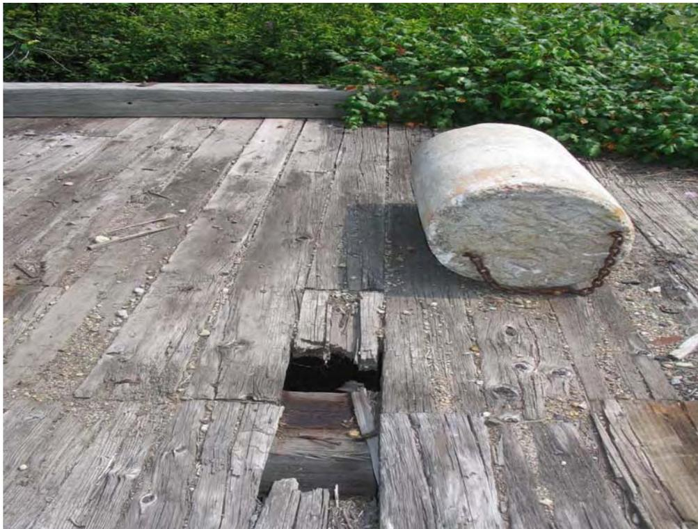
Picture 2: Broken wooden bridge over Rumford River
