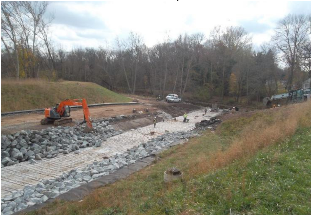
Photo #6 - Stream stabilization of Rose Valley
