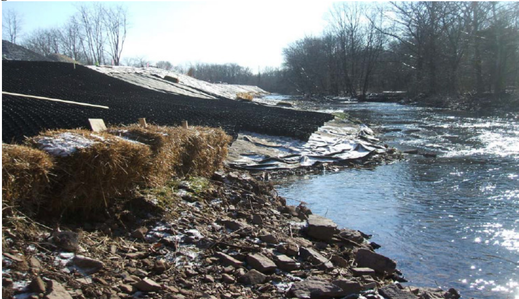
Photo# 3 - Stream bank stabilization of the Wissahickon Creek, with the geotextile fabric and geocells
