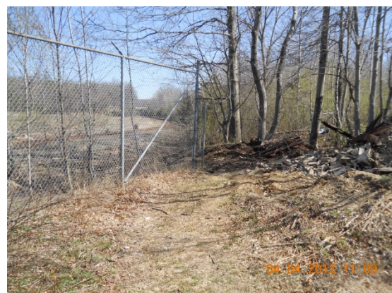
Missing portion of perimeter fence
