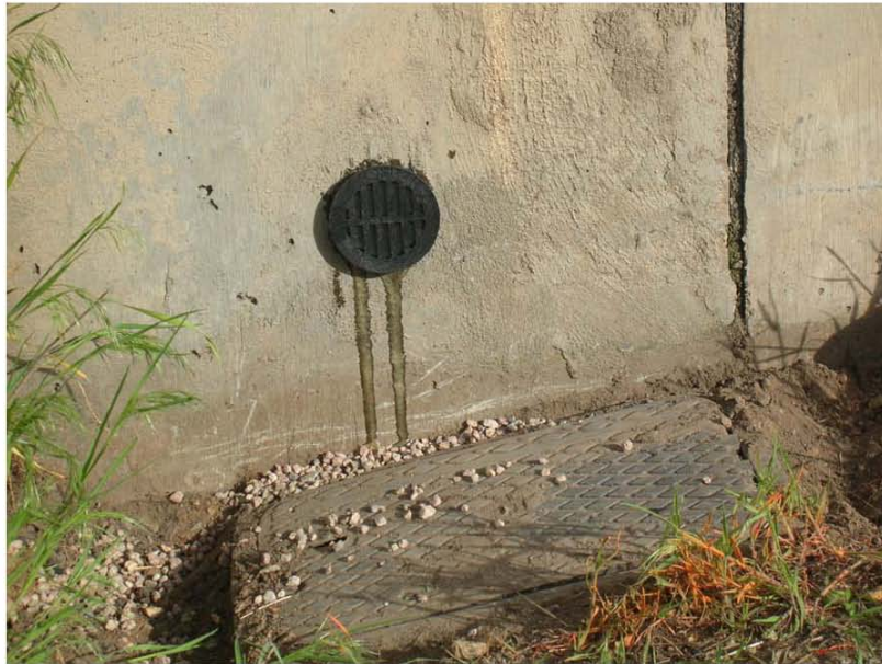
Figure 3. Photograph depicting hole-cover in retaining wall that needs to remain in place in order to prevent percolation of radioactive tailings materials onto the Durango Discovery Museum site.
