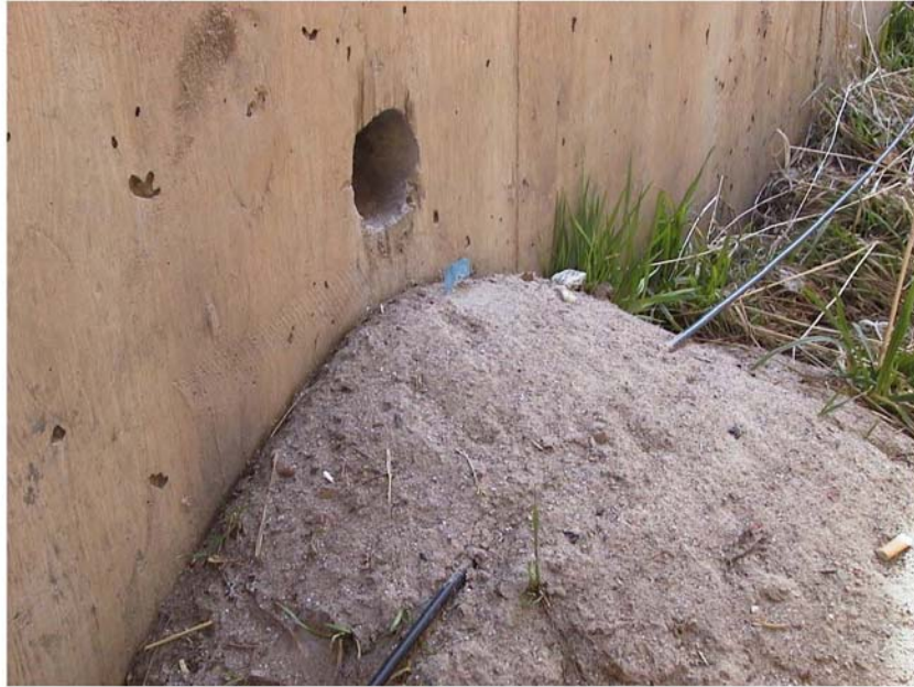
Figure 2. Photograph depicting hole in retaining wall that allows percolation of radioactive tailings materials onto the Durango Discovery Museum site
