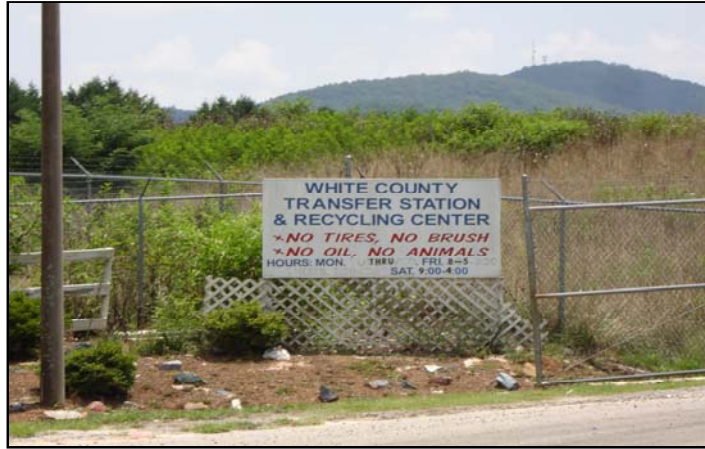
The White County Waste Transfer Station entrance is located in the Industrial Park adjacent to LHR Farms.
