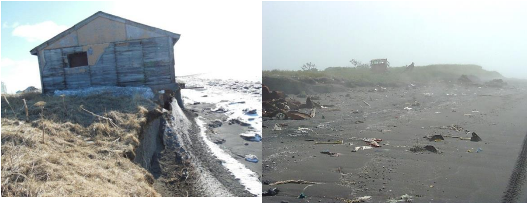
Figure 1 Erosion of shoreline revealing buried waste in seafood harvesting area
