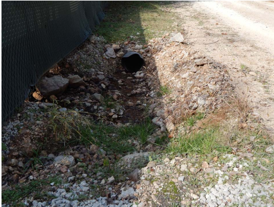
View of drainage ditch beside Arkwood Waste Water Treatment Plant.
