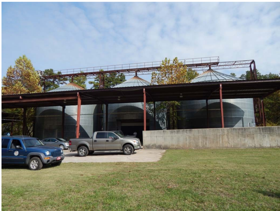
Front view of the empty treatment area with concrete slabs and three large silos adjacent to the railroad track. Contractors used this as work space while collecting samples.
