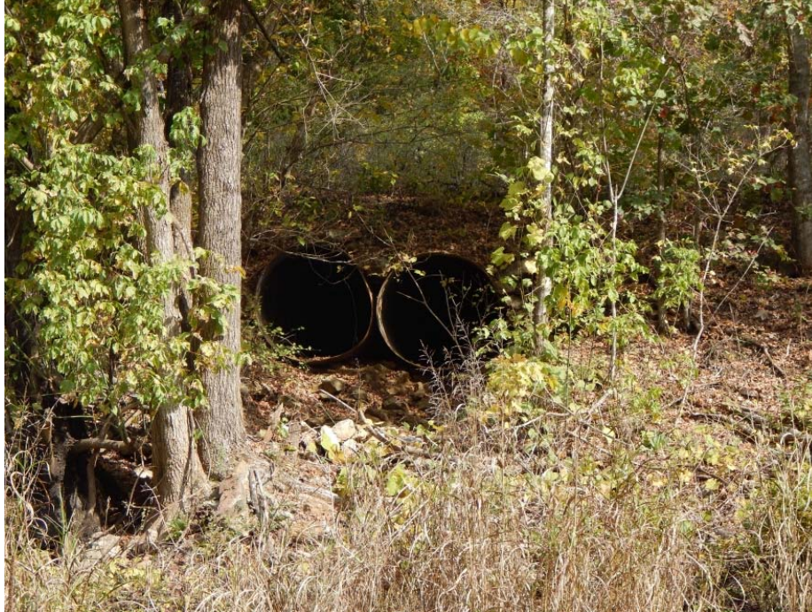
View of drainage discharge into New Cricket Spring off-site of Arkwood property.
