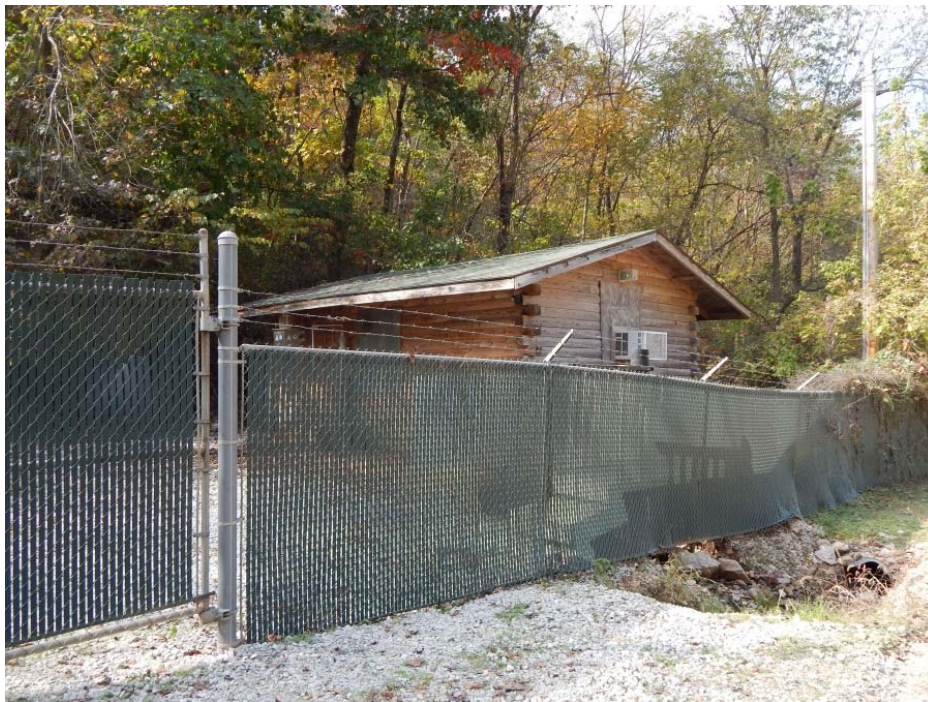
View of Arkwood Waste Water Treatment Plant (fenced and locked; not accessible to the public).
