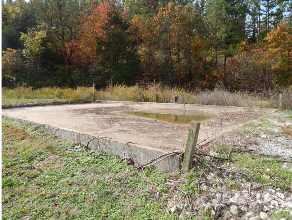
View of concrete foundation of the former decontamination pad.
