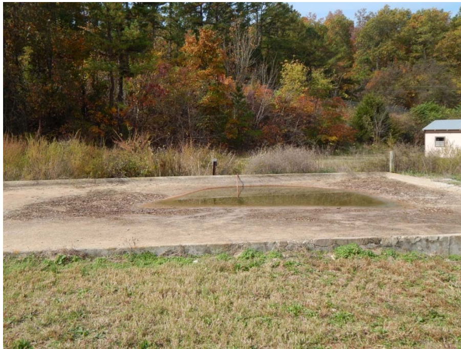
View of concrete foundation of the former decontamination pad (storage shed in background).
