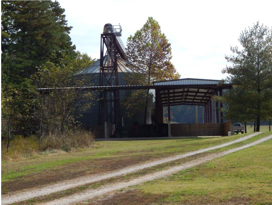
Side view of the empty treatment area with concrete slabs and three large silos adjacent to the railroad track.
