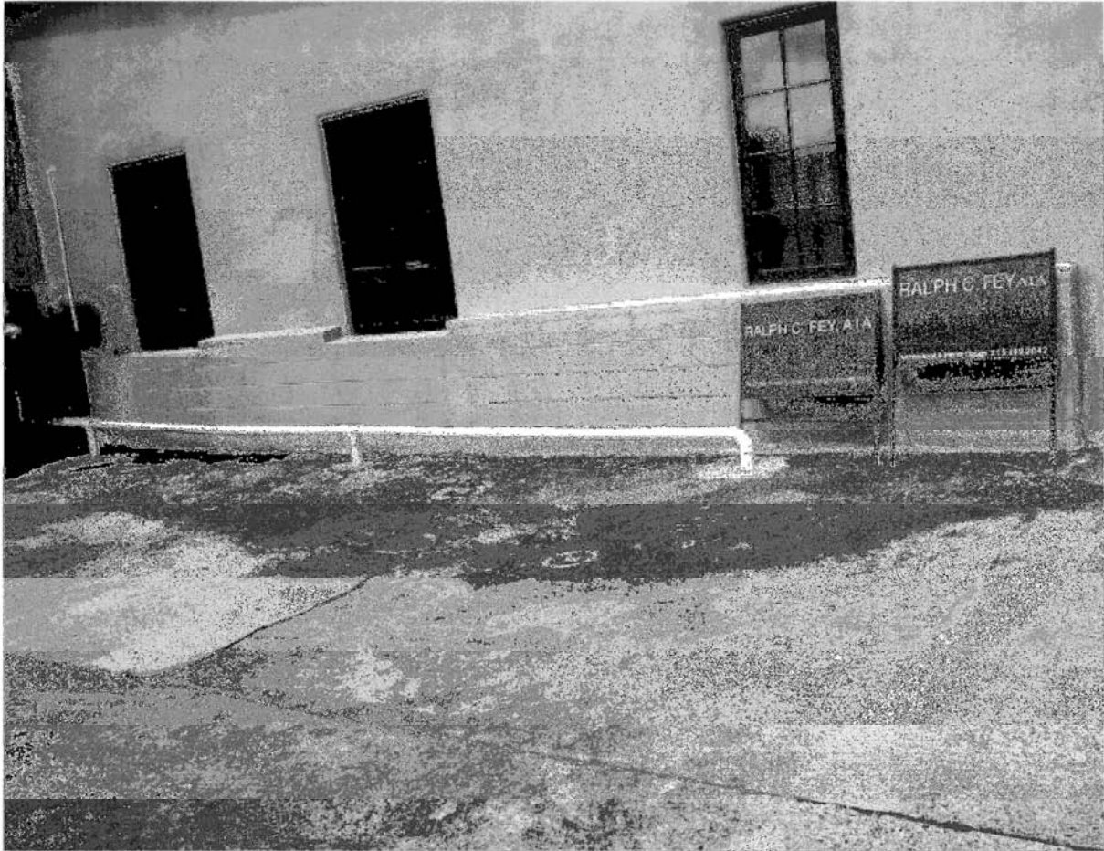
Figure 2. Picture of vapor mitigation system behind office 300, Chem Fab site
