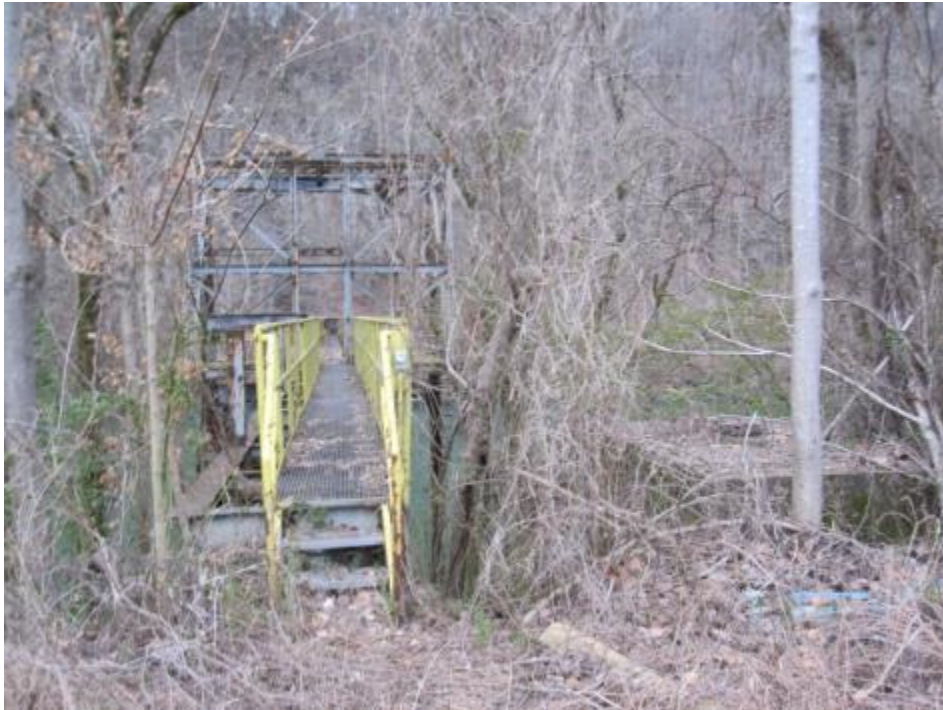
Photo 7 – Former walkway for a barge loading and unloading structure extending out over the Emory River. This physical hazard is unfenced and is open for trespassing. (Photo credit: Brad Parman, 03/11/13).
