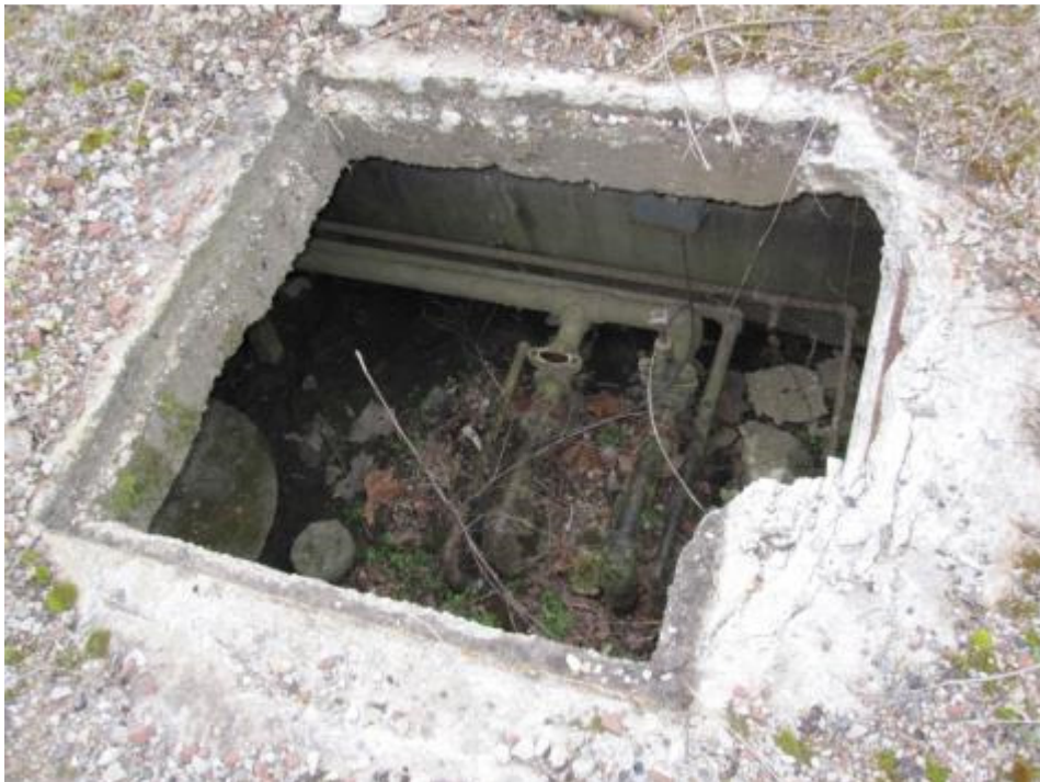
Photo 8 - Open former hydraulic oil underground storage tank (UST), one of the several open pits across the former manufacturing area of the site. Note the extensive piping and valves within the UST. The UST access is uncovered. (Photo credit: Brad Parman, 03/11/13).
