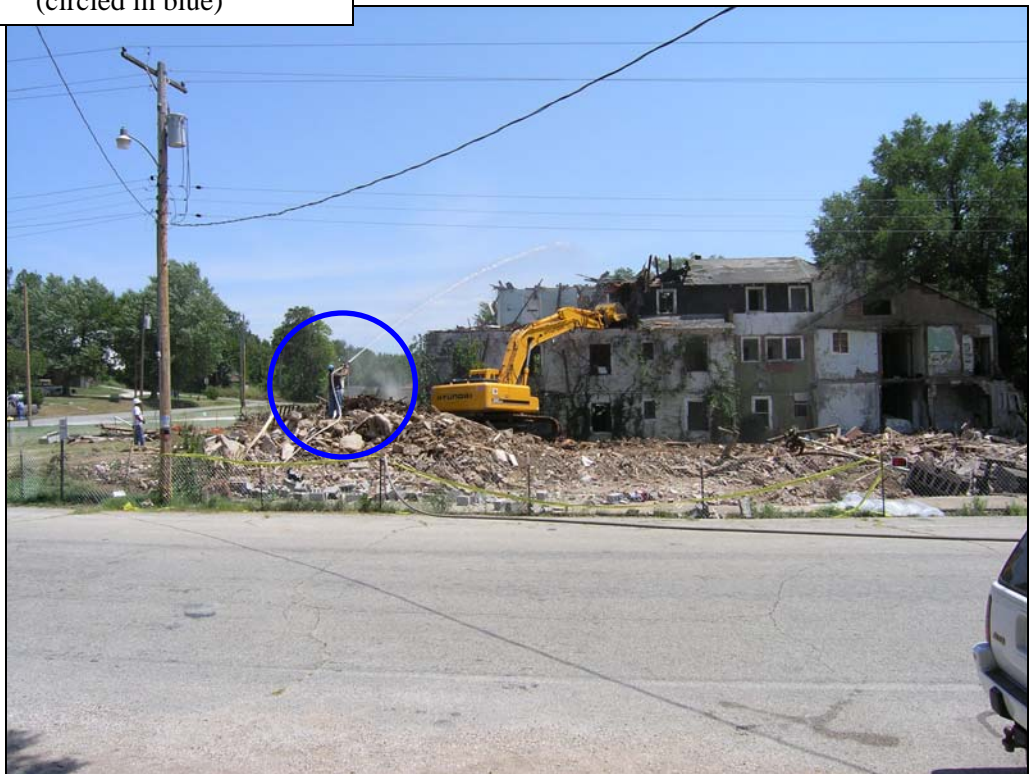
Cardwell Hospital Site, Dust suppression application. (circled in blue)
