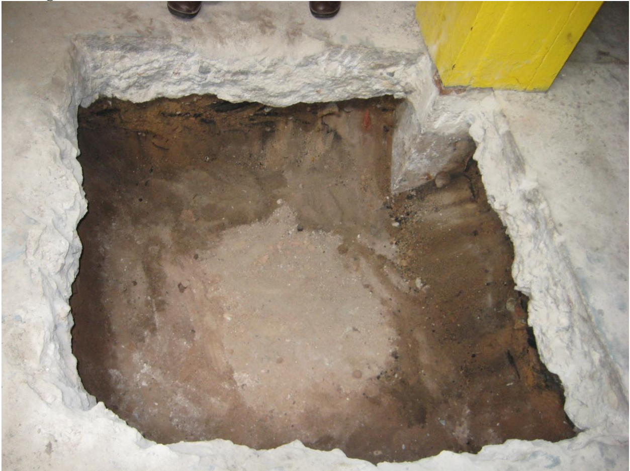
Figure B.7. Subsurface and concrete excavation around pylon within building (note soil staining)
