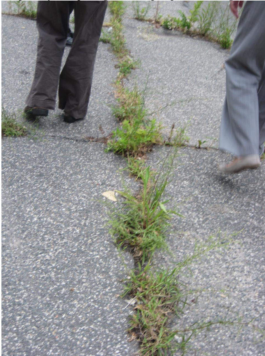
Figure B.2. Concrete cover outside the building (vegetation that penetrates the concrete show a possible pathway for vapor migration and precipitation recharge)
