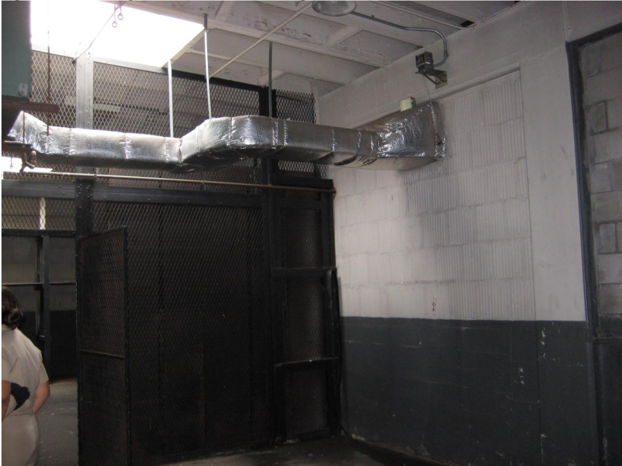
Figure B.9. Existing ductwork in the building on-site
