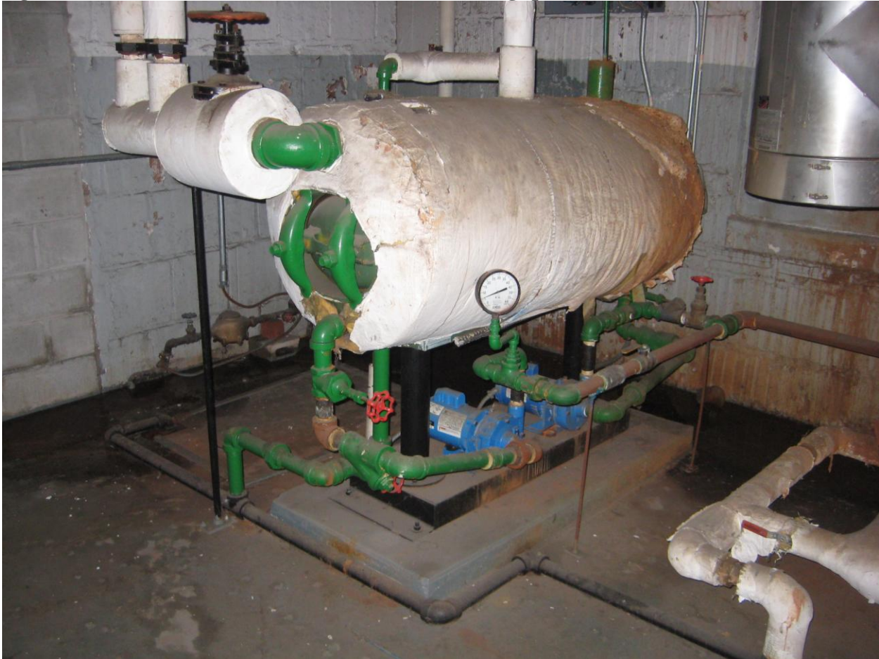
Figure B.5. Old insulation material inside the building (potential asbestos source)
