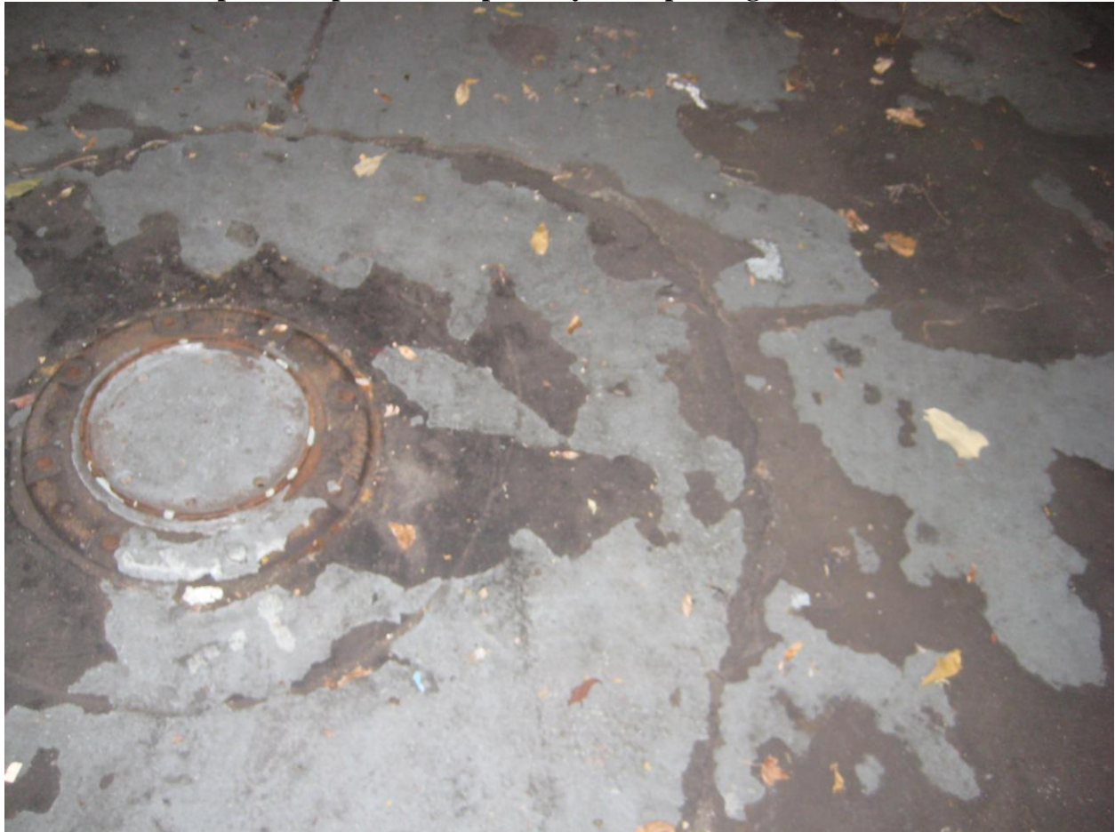
Figure B.3. Concrete flooring with manhole inside the building (structures that span the concrete can be a potential preferential pathway for vapor migration)
