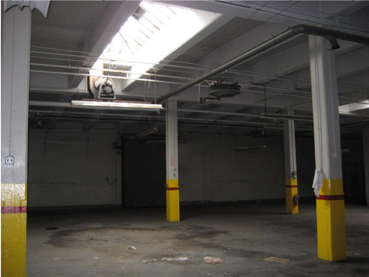
Figure B.4. Fluorescent lighting ballasts and staining of concrete flooring inside building
