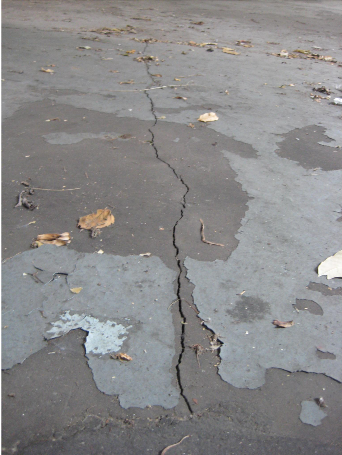
Figure B.1. Concrete flooring inside the building (cracks can be a potential preferential pathway for vapor migration)
