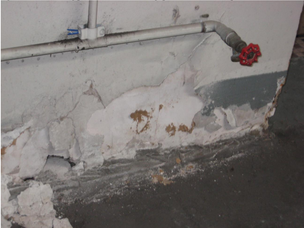
Figure B.8. Crumbling paint inside the building (potential lead based paint source)
