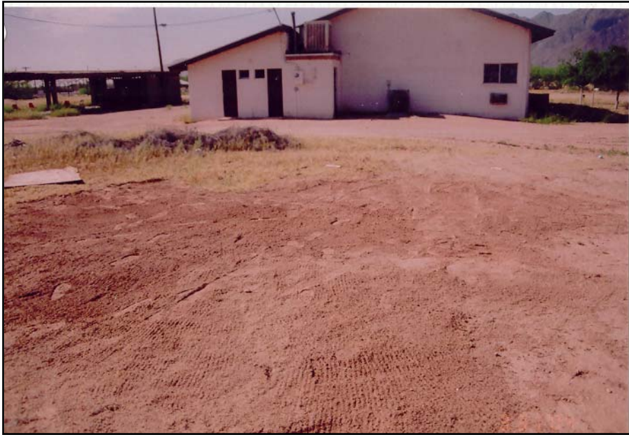
Figure 7: Remediated area located behind the Gila Crossing Presbyterian Church
