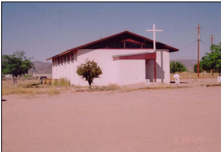
Figure 2: District Six Gila Crossing Presbyterian Church, Main Entrance (before and after exterior remediation)
