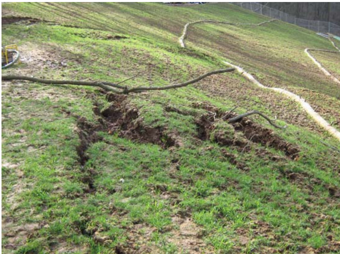
Figure 6. Heizer Creek Landfill Site after Rain Storms in March 2009 (Sloughed Area)
