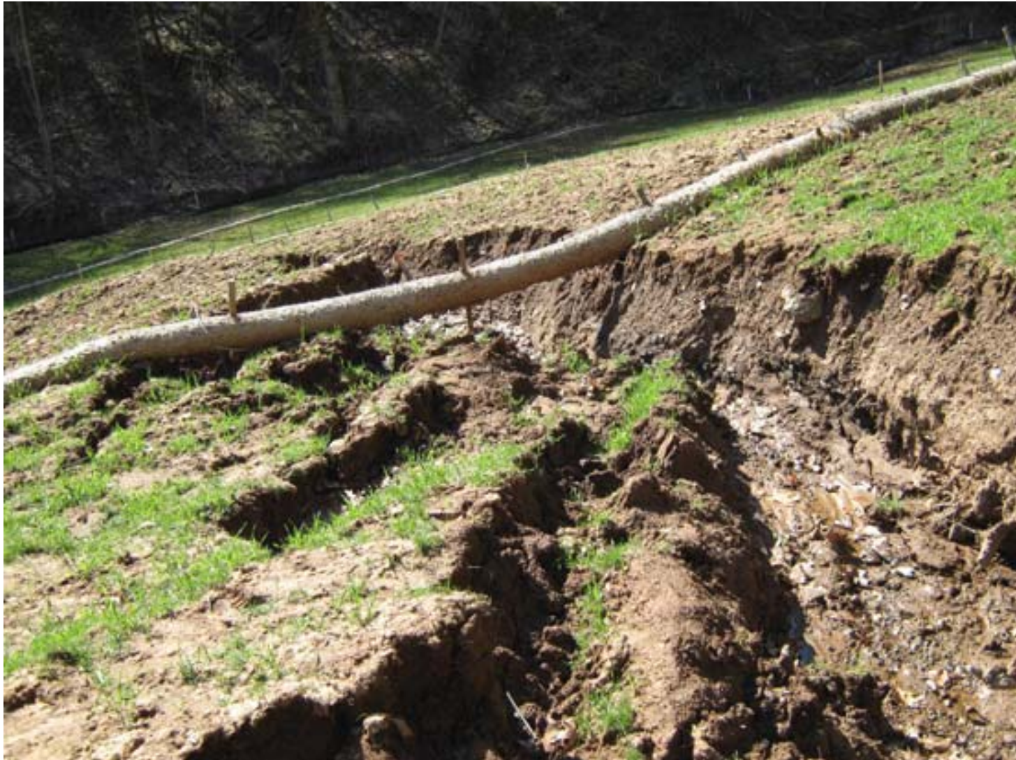
Figure 7. Heizer Creek Landfill Site after Rain Storms in March 2009 (Northern End of Slip – Erosion Channel)
