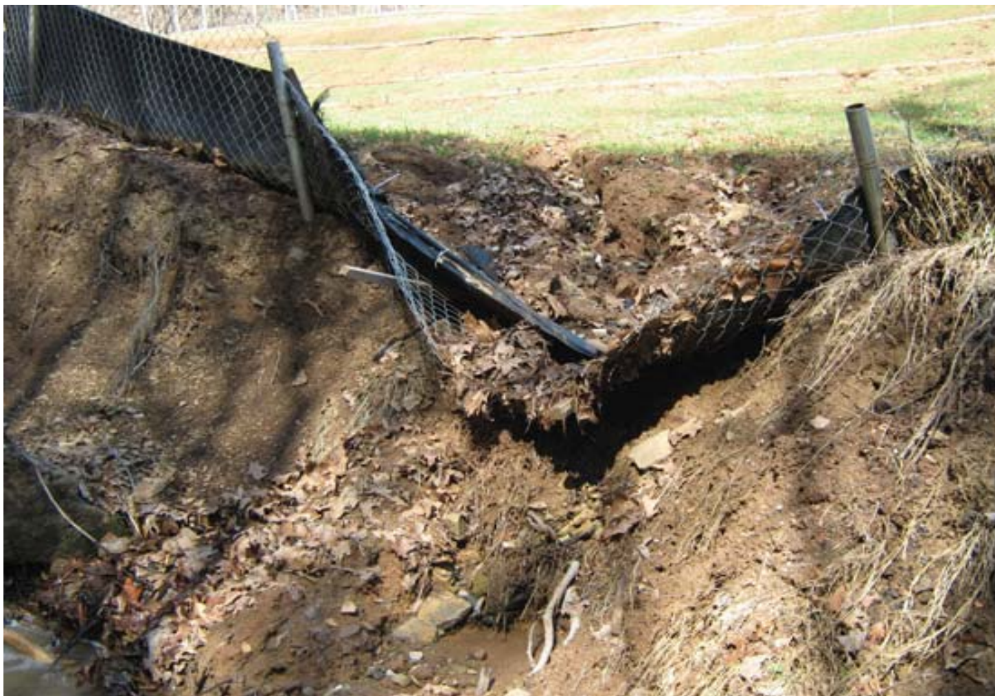
Figure 8. Heizer Creek Landfill Site after Rain Storms in March 2009 (Silt Fence near the End of the Diversion Ditch on the Southwest area of the Site)
