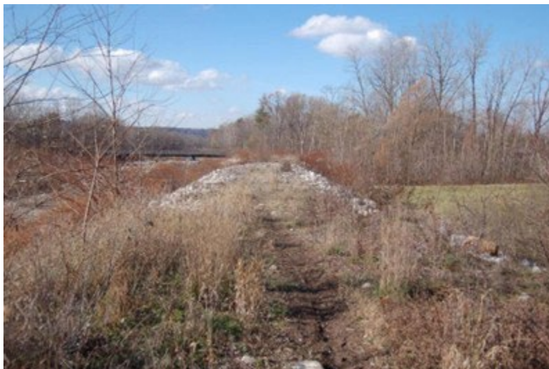
Figure 2. Earthen Berm at Rear (South) of Jard Site (2017)
