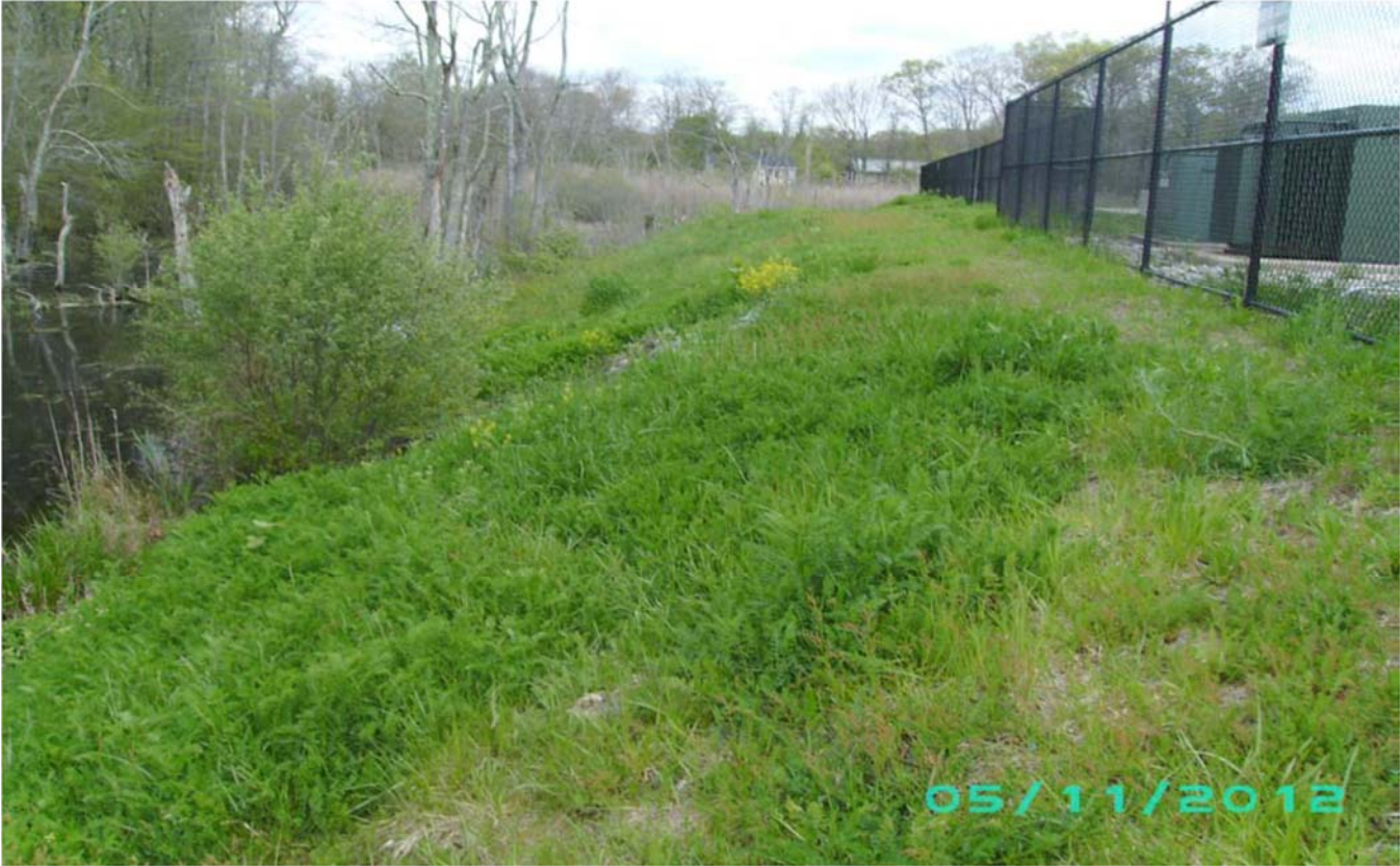
Figure 3. Stabilized slope along northwestern slope looking north
