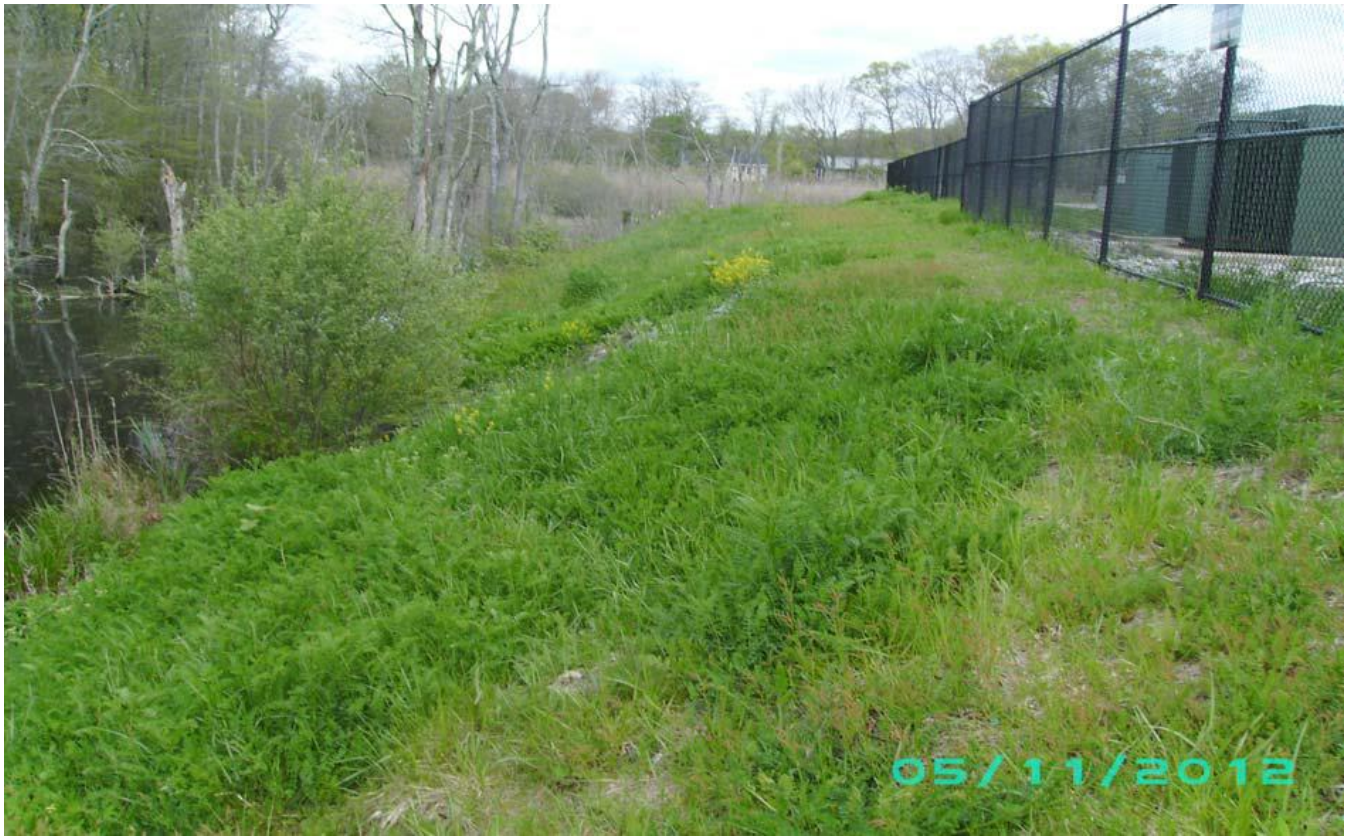
Figure 3. Stabilized slope along northwestern slope looking north
