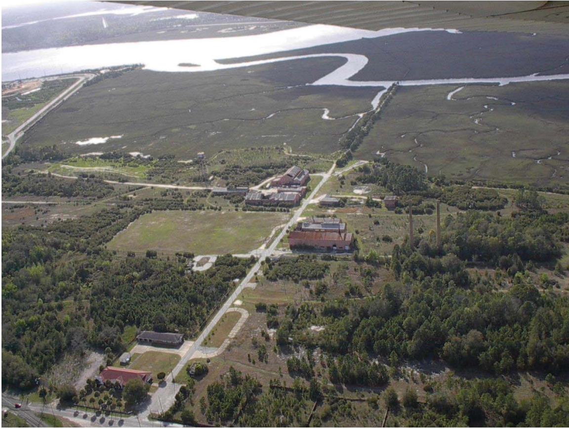
Figure A2. Site Map Showing Current Onsite Structures on Dry-land Area with Marsh in Background (March 2004)
