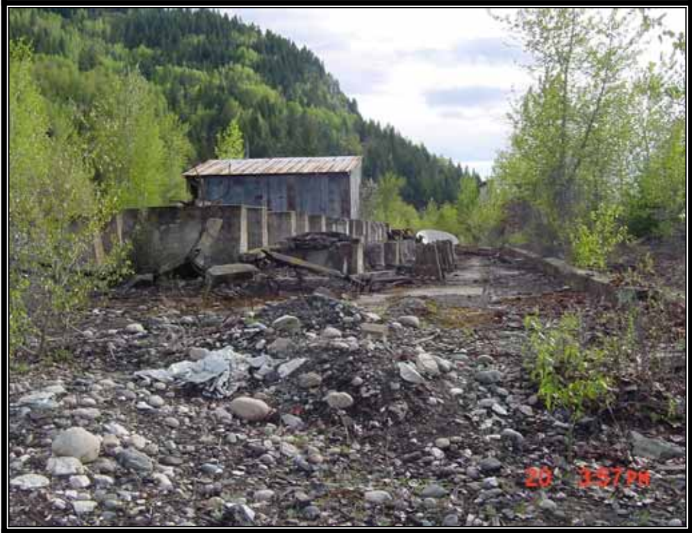
Photo 4. Remaining foundation on-site
