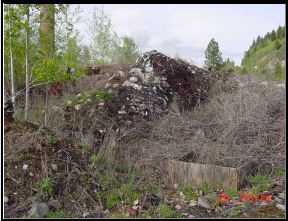
Photo 3. Remaining foundation on-site
