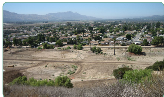
Photo of the Pacific Coast Pipeline Superfund site, looking west, September 2012.
