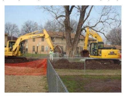
View of two excavators used to excavate soil and load disposal trucks at Redwood Early Childhood Center.
