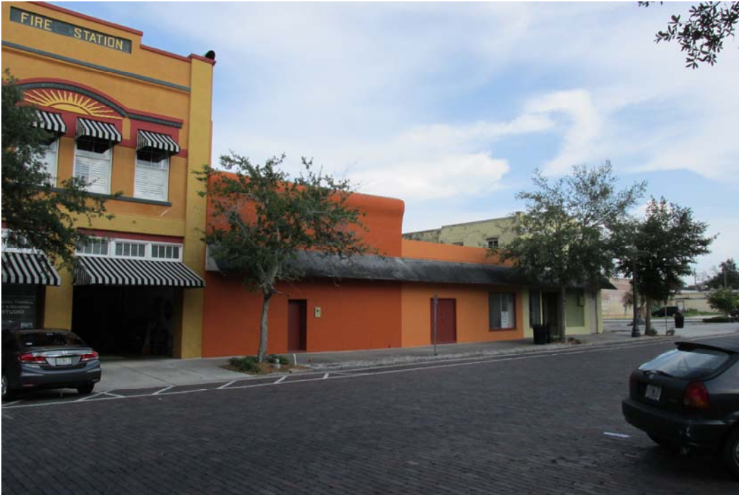
Photograph 1. Front of the site (three low buildings) in 2013.
