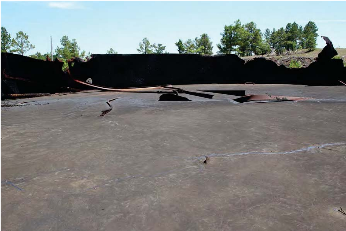
Photo 19: Cut down former asphalt tank with flowable asphalt bottoms near Industrial Area. 2016
