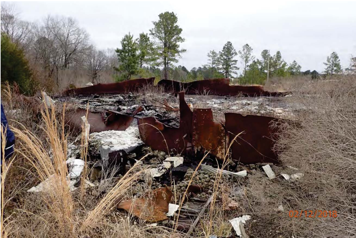
Photo 23: Cut down former asphalt tank with flowable asphalt bottoms near Industrial Area. 2018
