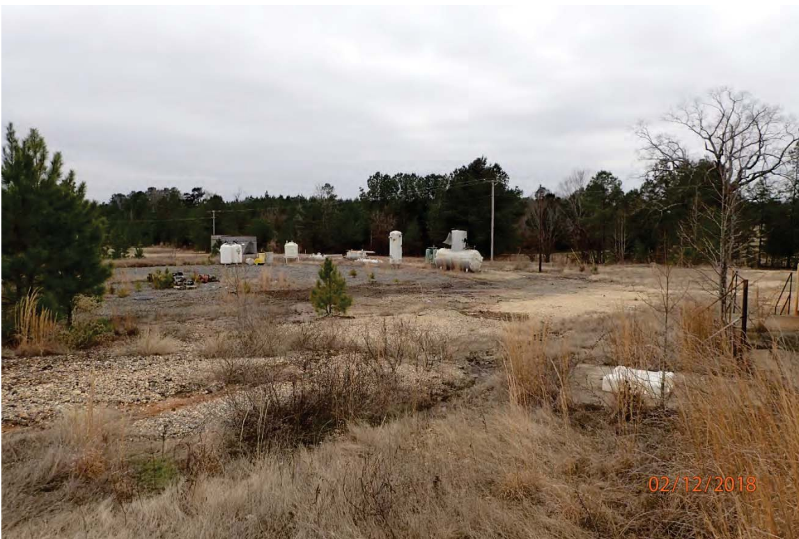
Photo 8: Tanks and former equipment at Industrial Area. 2018
