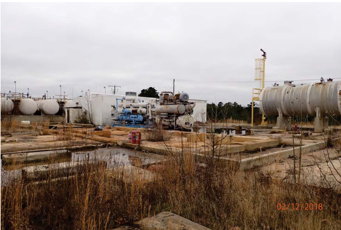
Photo 6: Tanks and former equipment at Industrial Area. 2018
