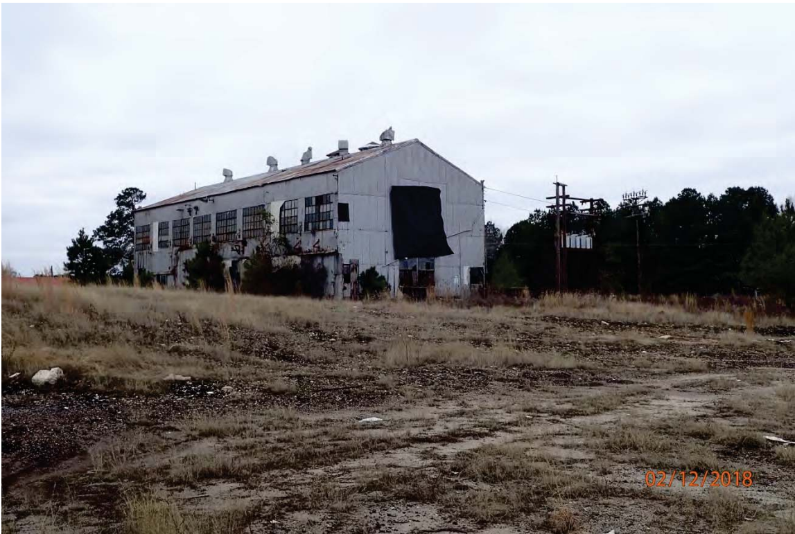
Photo 25: Unsecured boiler house near Industrial Area. 2018
