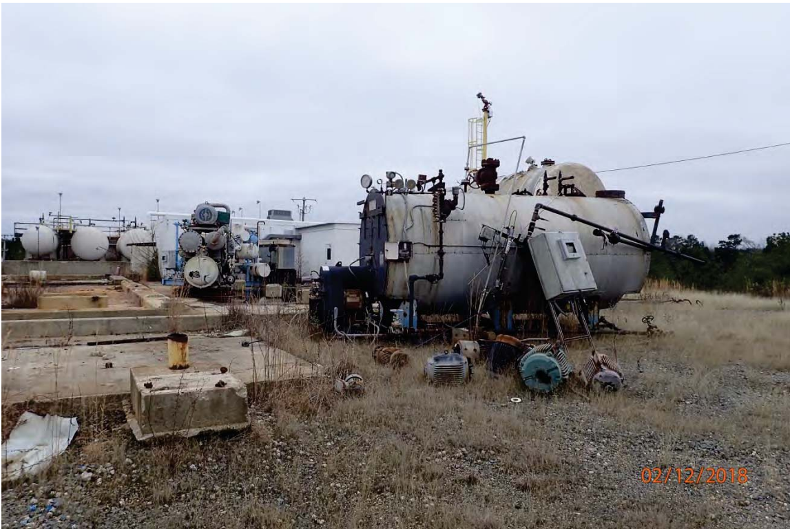
Photo 7: Tanks and former equipment at Industrial Area. 2018
