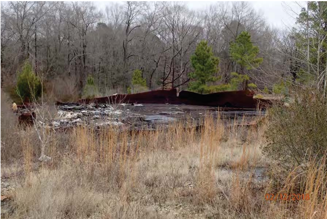
Photo 17: Cut down former asphalt tank with flowable asphalt bottoms near Industrial Area. 2018
