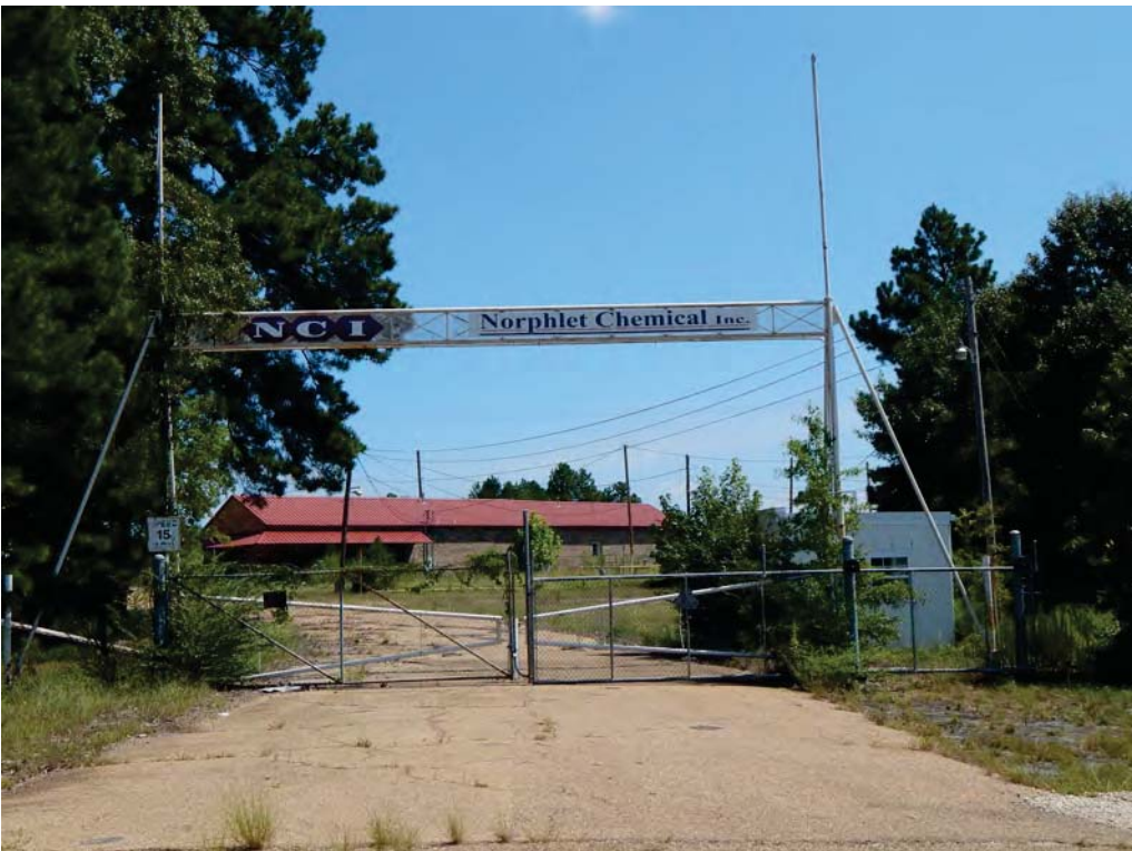
Photo 4: MacMillan Road Gate. 2014
