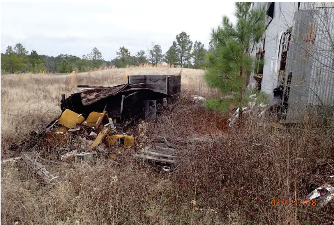
Photo 12: Debris adjacent to the boiler house near Industrial Area. 2018
