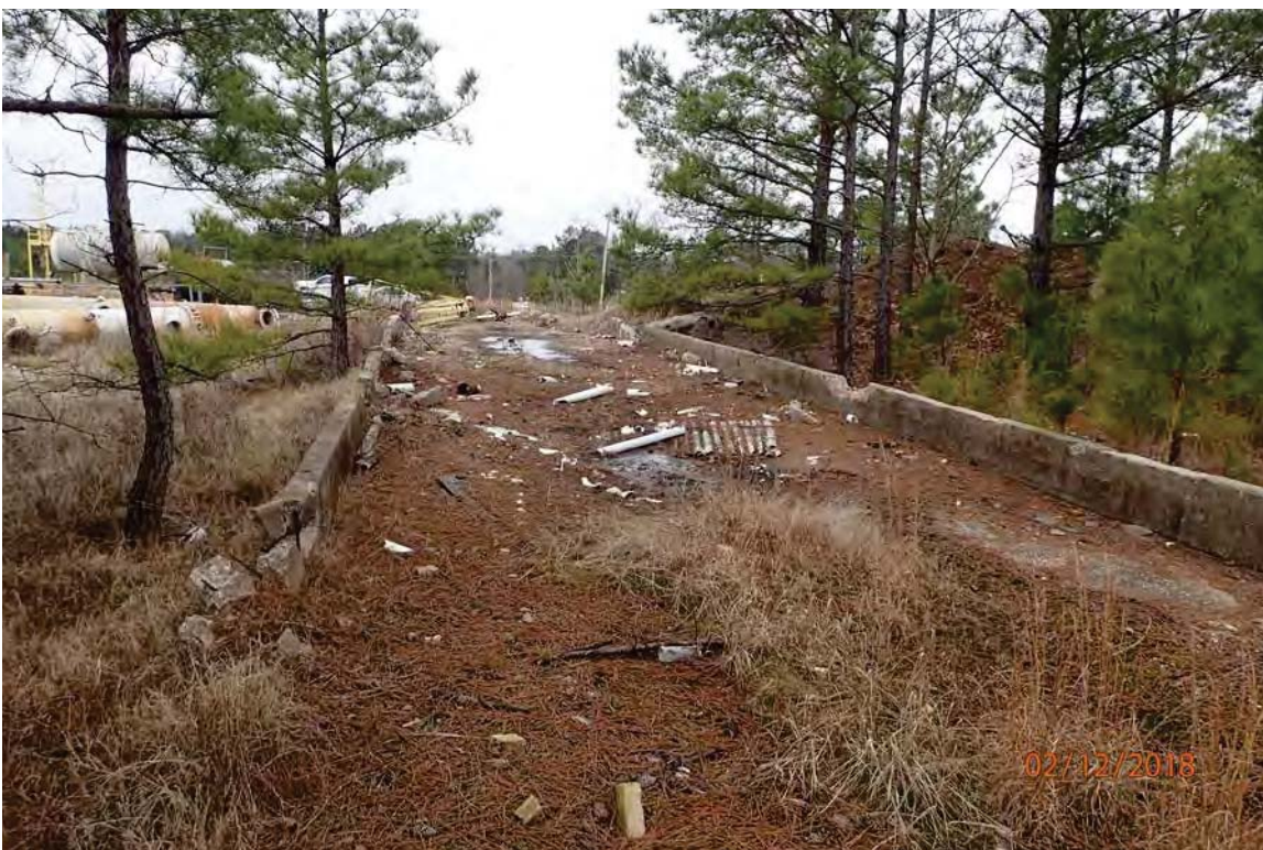
Photo 10: Debris near Industrial Area. 2018
