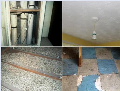
Avoid touching or disturbing any possible asbestos-containing materials in your home. Pictures clockwise show examples of old pipe insulation, textured ceilings, damaged floor tiles, and vermiculite attic insulation.
