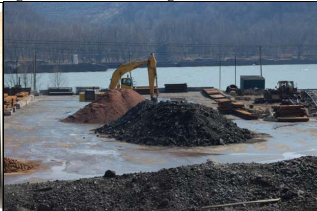
Figure 2: Outdoor storage areas -
