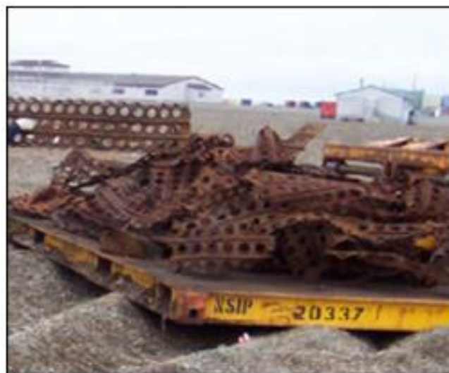
Figure 2: Marston matting removed from Site 6
