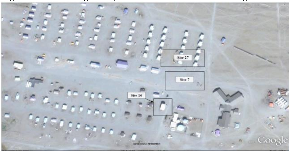
Figure 7. Area Showing Sites 7, 16 and 27 near Homes and Buildings
