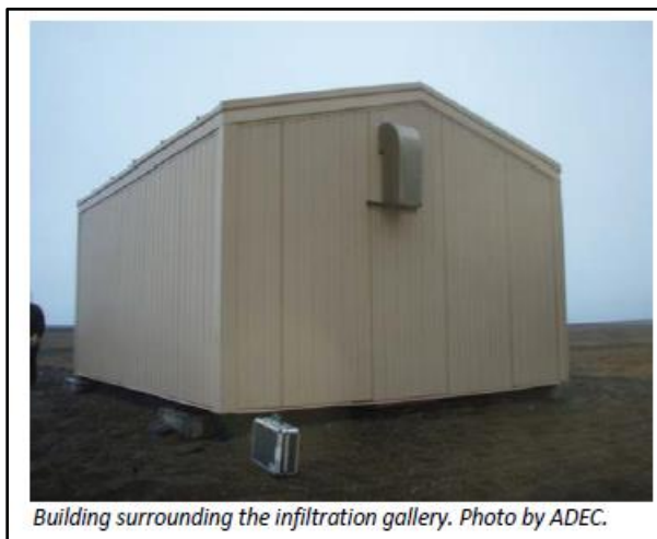
Figure 4. Infiltration Gallery Building
