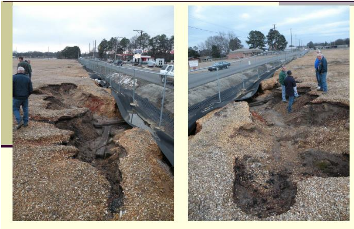
Photo 3. Erosion Along 14 th Avenue
