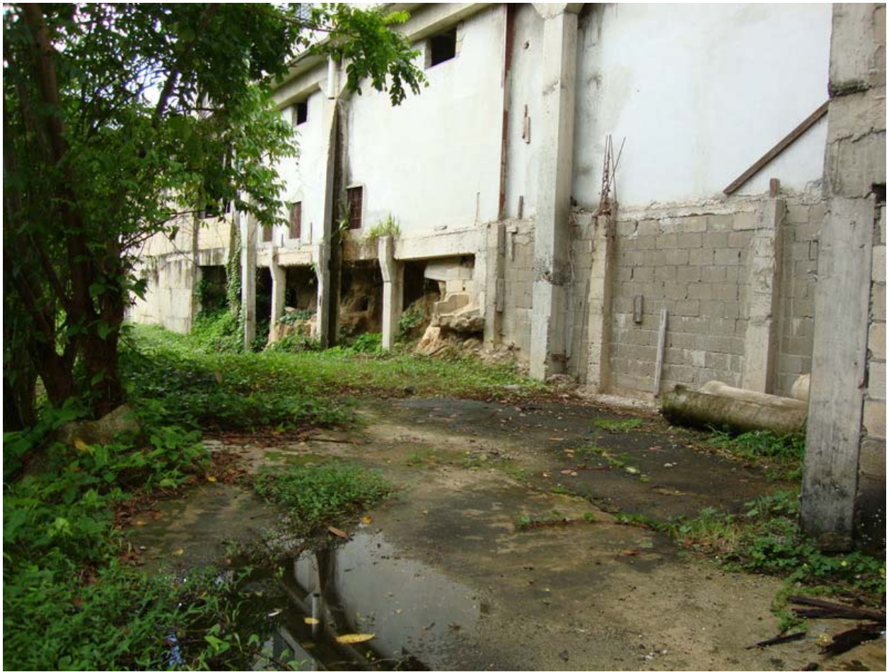
Southwest wall of the PPI building which faces the Vivi River
