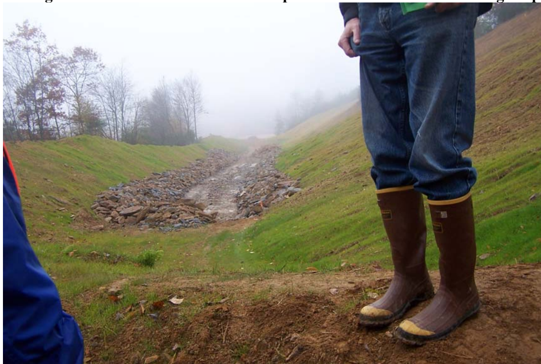
Figure 15. Ore Knob Mine NPL site, October 2009. View of channel under construction re-routing stream around outside northwest perimeter of 20-acre main tailings impoundment.
