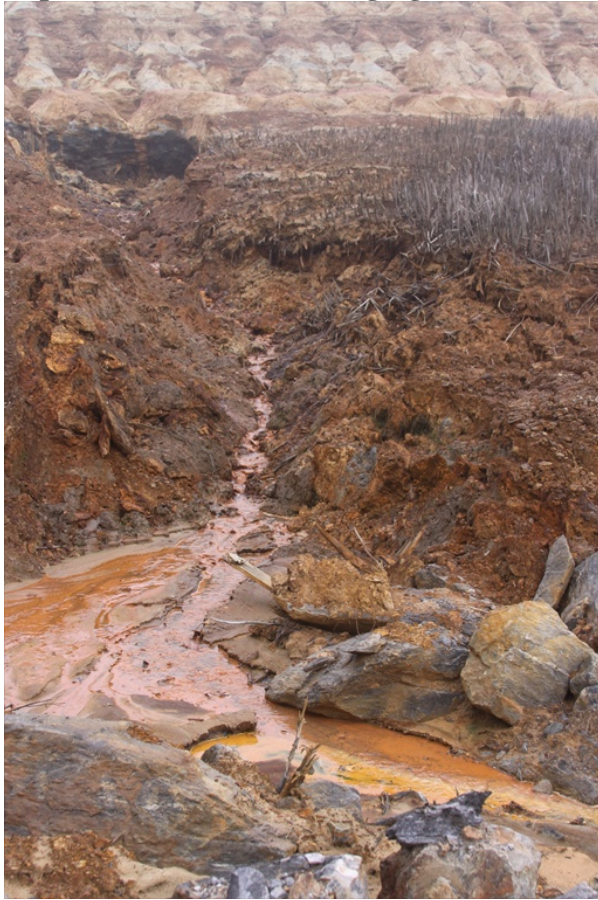
Figure 12. Ore Knob Mine NPL site, October 2009. Water discharging from face of tailings impoundment dam around area of 24-inch pipe carrying surface water under the impoundment and discharging at the base of the dam.
