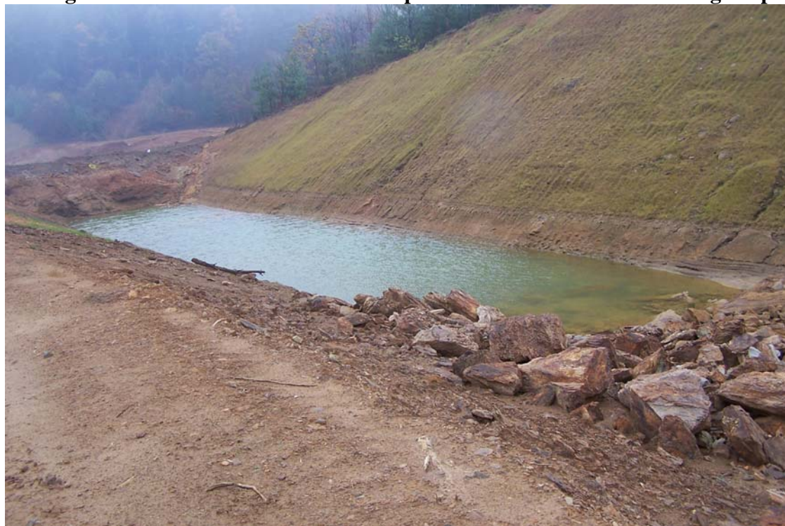
Figure 16. Ore Knob Mine NPL site, October 2009. View of channel under construction re-routing stream around outside southwest perimeter of 20-acre main tailings impoundment.
