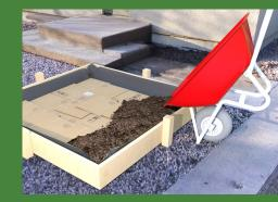
c. Finally, fill the bed with clean soil and use a garden rake to level it out.
