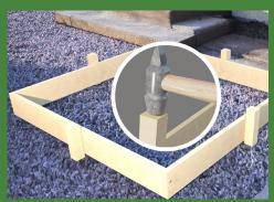
d. Pound 2x2 wooden stakes into the ground around the outside of the frame to reinforce sides.
