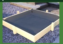
a. Cover the spot for your raised bed with landscape fabric, using enough to extend a little beyond the frame edges to help protect the wood from rotting.
