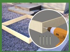
c. Fasten the boards with four screws at each corner.
