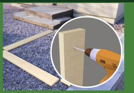
b. Pre-drill holes (to keep the wood from splitting).
